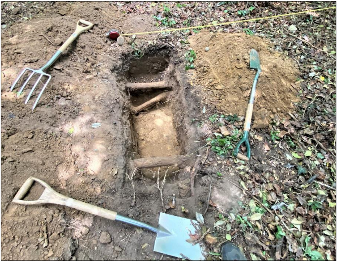
Figure 4: Excavated trench down to about 50cm depth showing three roots about 7–10cm in diameter.
