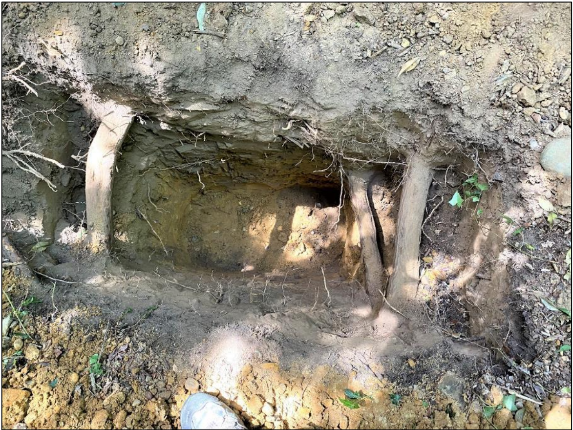
Figure 6: Trench excavated down to about 1m depth showing obvious smaller roots at the bottom with species characteristics associated with T184.
